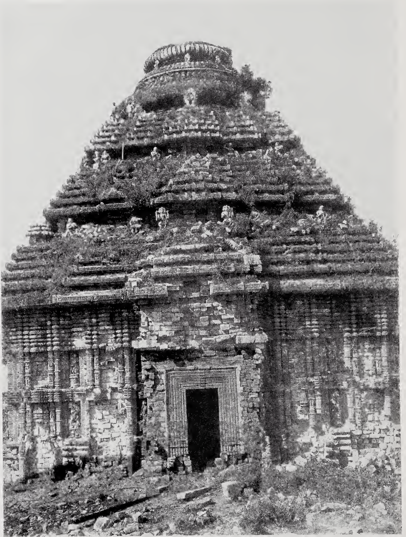
Jagamohana, before repair, view from east, ASI.
